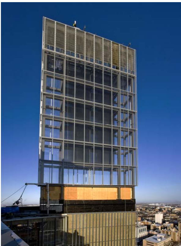
Fig 9: Solar Chimney, Detail, under construction
