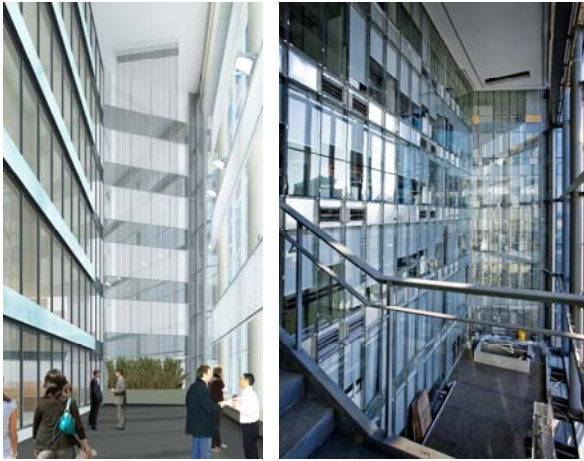
Fig 8: Wintergarden, Rendering (left) and under construction (right)
