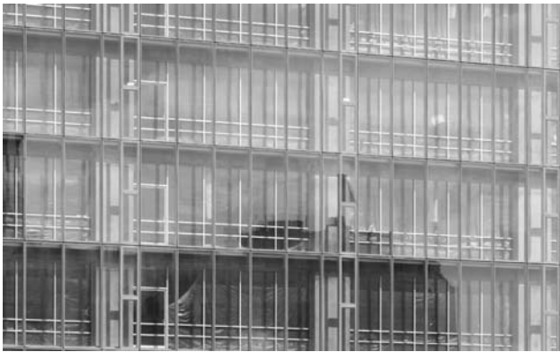
Fig 11 Detail of double-façade
